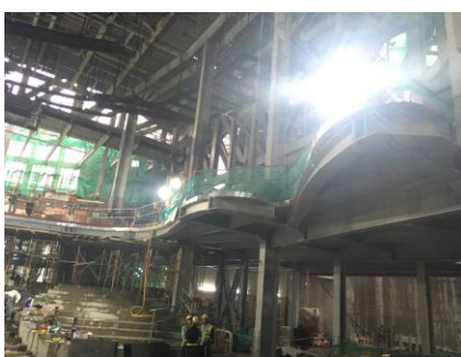
Fig. 2. The external façades and internal steel structure of Xiqu Centre.
