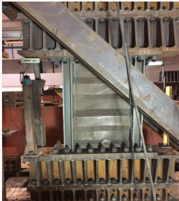
Fig. 20. Buckling of S1 at drift ratio of 1/75
