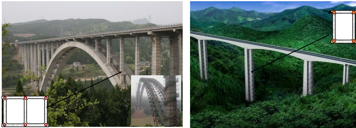
(a) Zhaohua Jialing River Bridge
