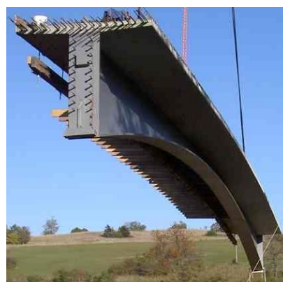
Fig. 1. Prefabricated composite bridge girder with horizontally lying studs [2],[3]
