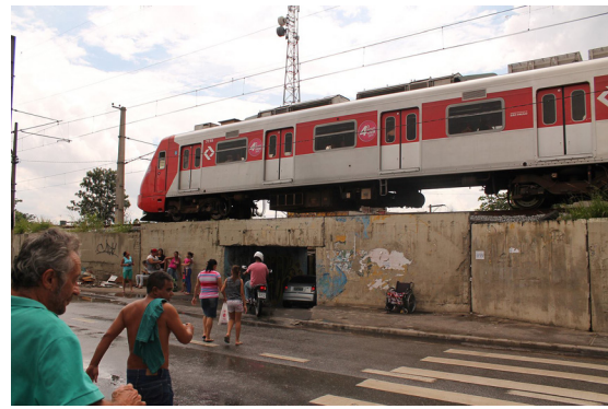
Figure 2. Wormhole: the tunnel that crosses the railroad (Leonardo Gobbi, 2016)
