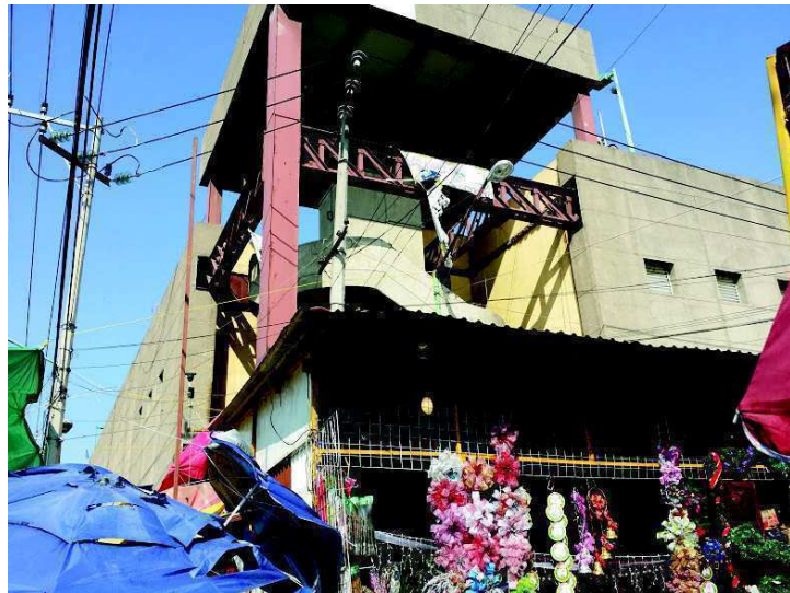
Figure 3. Plaza 2000 Merced in Mexico raised as demolition in the rescue Project
