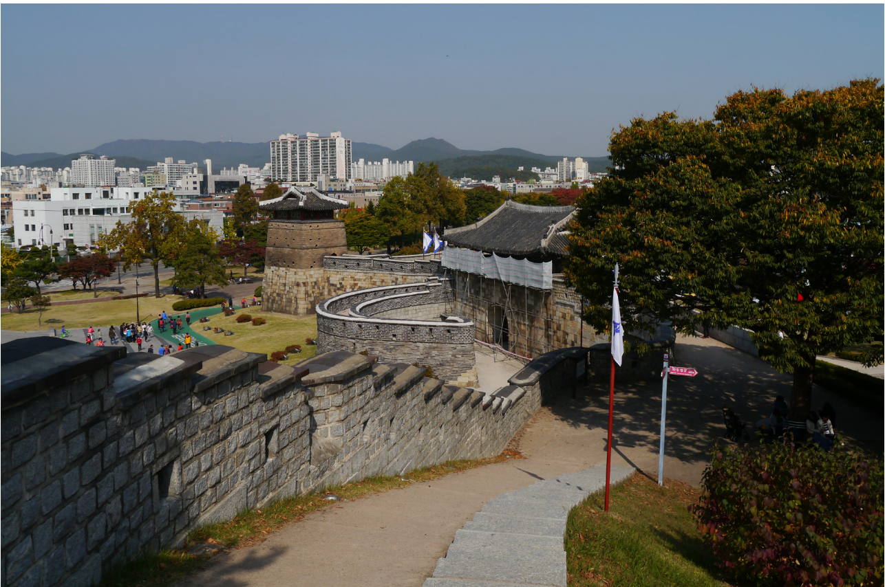
Figure 2. Preserving the fabric at Suwon fortress, South Korea .
