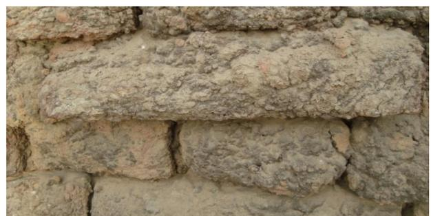
*Fig. 19 The penetration of the water vapour, and expansion, inside the pour.*
