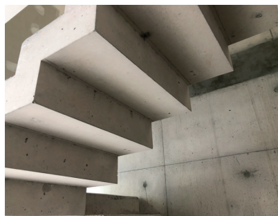
Figure 10. Details of the texture of the exposed concrete. 2019. sanahuja&partners. ©Pablo Morán / Figura 10. Detalles de la textura del hormigón visto. sanahuja&partners. 2019. ©Pablo Morán.
