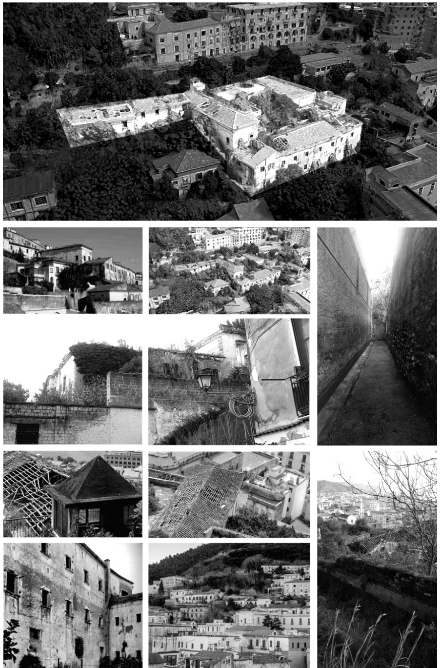
Figure 7. Current state of the Convent of San Francesco d'Assisi (photos by authors).
