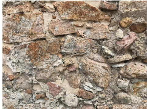
Fig. 8. Stone irregular ashlars of north side tower wall.
