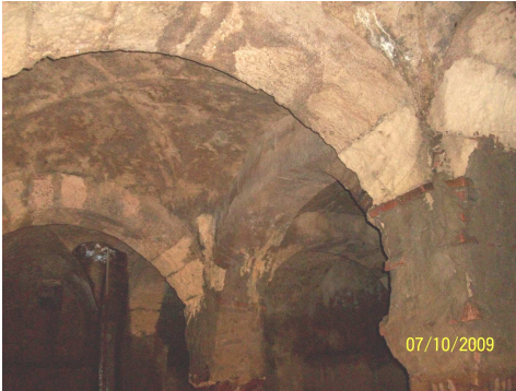
Fig. 5. Vaults covering the medieval cistern (AUA photography, Annaba, 2009).
