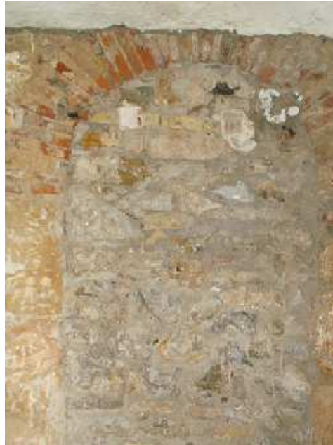
Fig. 7: Ribat: original arched opening built in stones obstructed in the nineteenth century.
