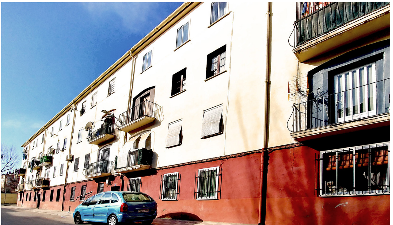
Figure 3 and 4 | Original and Current status 64 dwellings Albacete, RENFE, 1952. (AHF-FV-0033 -Own archive).
