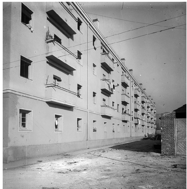
Figure 6 | RENFE, 224 subsidised housing in Madrid-Delicias, 1954. (AHF-ADC-0180).
