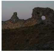
Ruina de Cañavate - vista general
