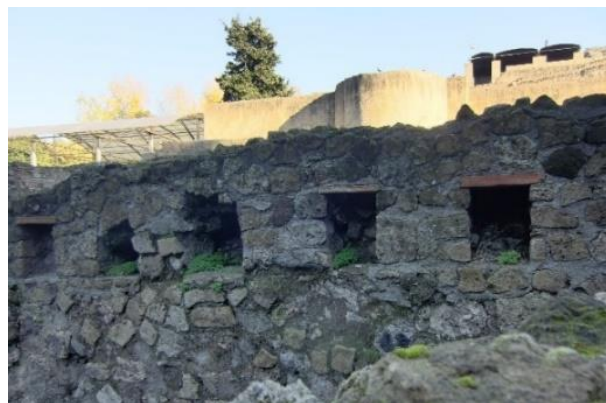
Figure 2: Sockets left by floor joists in a wall, Pompeii.
