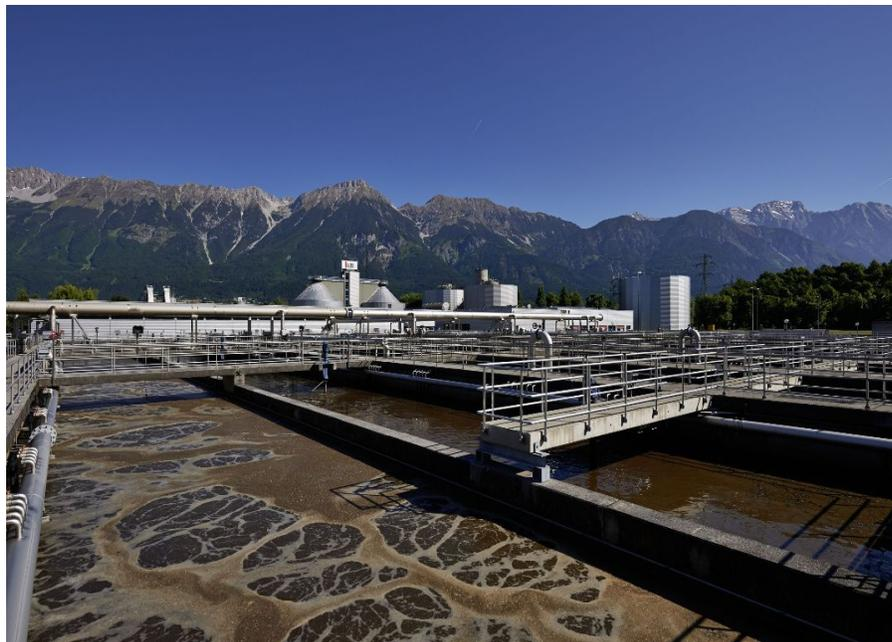
Figure 6 – Sedimentation tank in a purification plant ([https://www.bmlrt.gv.at/fotoservice/wasser/abwasserwirtschaft/IKB\\_6205\\_bah.html](https://www.bmlrt.gv.at/fotoservice/wasser/abwasserwirtschaft/IKB_6205_bah.html), with kind permission of the BMLRT, Austria).
