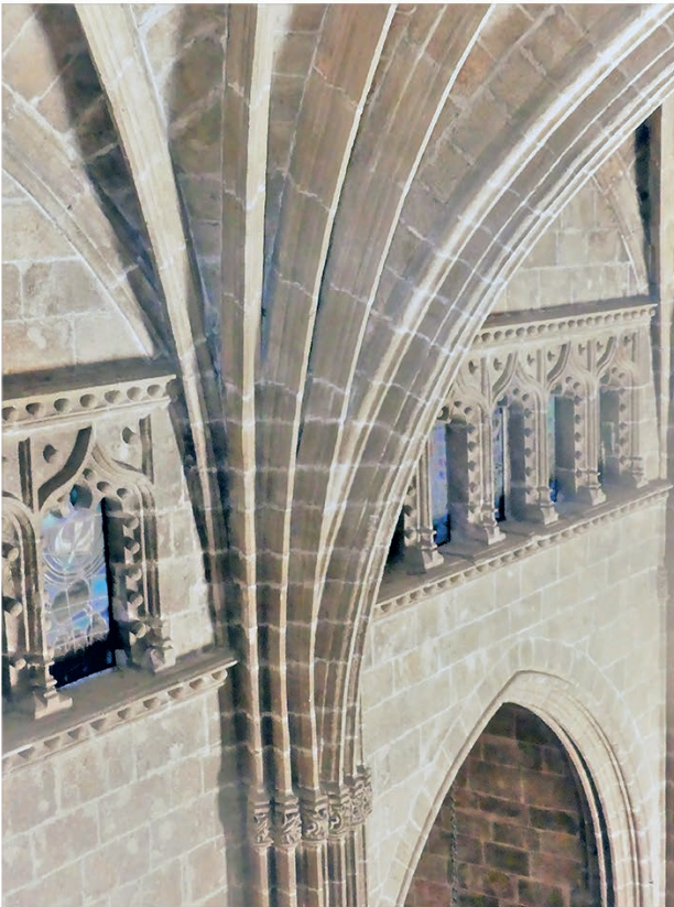
Fig. 20. View of starred vaults of the church of San Bartolomé in Jávea during a 3d laser scan and a detail of the tas-de-charge where the arrangement of the ribs can be seen. (Source: Capilla, Esther, 2021).
