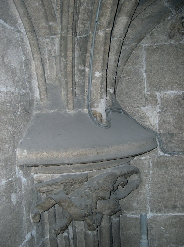
Fig. 4. Detail photograph of the spring corbel and the ribs that come out of it. (Source: Capilla, Esther, 2004).
