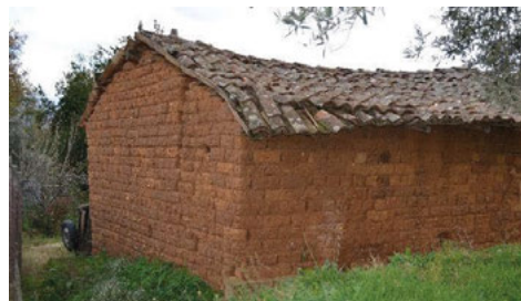
Fig. 4. District Iotta: house with raw clay bricks.
