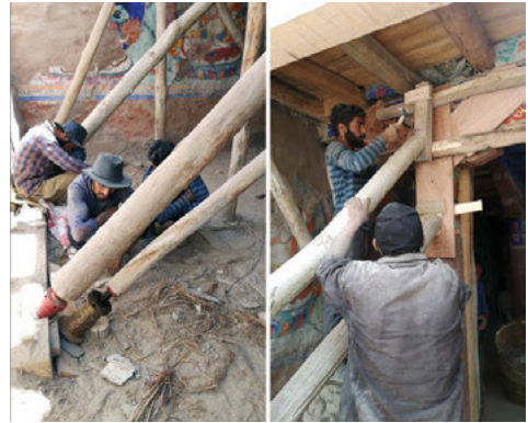
Fig. 15-16. Installation of the props with hydraulic jacks (left). Fixing a temporary load distribution timber frame on the columns and beams (right).
