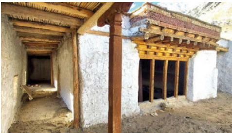
Fig. 21. The terrace. Image credit: Javed Hanif architect.
