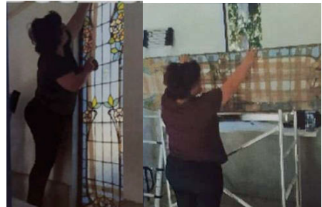
Fig. 8. Disassembly works. British Cemetery (Source: Benavent, 2017).
