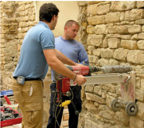
Fig. 7. Detail of the process of extracting the stone from a load-bearing wall to analyse its internal composition. It is possible to observe that the wall is without mortar but just a mud poor in lime. (Source: Millán, 2014).
