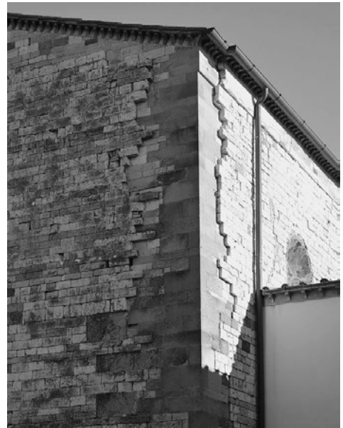
Fig. 3. damage to the wall caused by the earthquake in 1542. Church of Sant'Agata, Mugello (Source: Bordoni, 2021).
