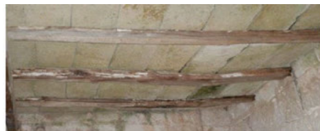
Fig. 11. Timber floor with timpagnoli (Source: Mami, 2018)
