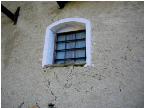
Fig. 9. Sketch of the plaster survey (Arvier) and example of plaster (Allein).
