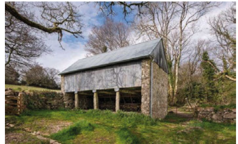
Fig. 1. Beckhams Linhay. East elevation following repairs (Source: Copyright Historic England Archive, Davies, 2021).
