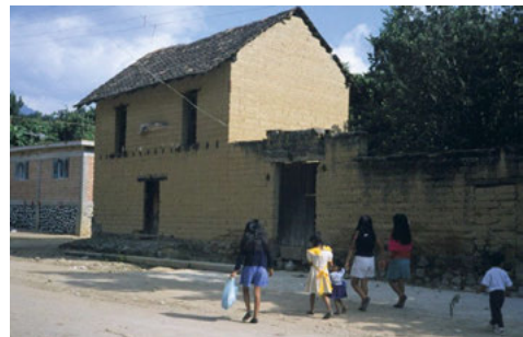
Fig. 3. Adobe house in Hueyapan (Source: Aguilar Prieto, 2001).
