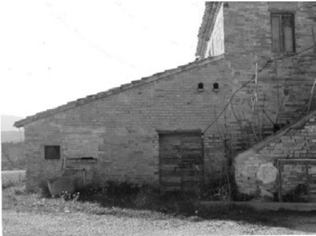
Fig. 8. Transformations of farmhouses. The construction of a new added volume changed the façade in the relation with the road (Source: Cipolletti & Guaiani, 2022).
