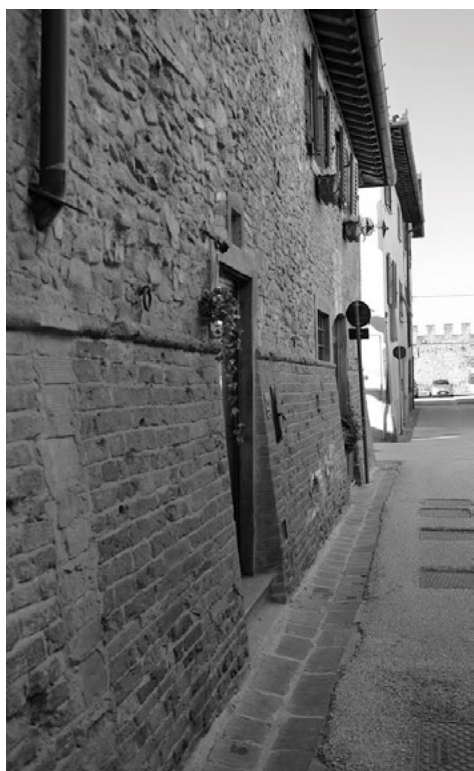
Fig. 1. Reinforcement wall of a house in Scarperia (Source: Bordoni P., 2021)
