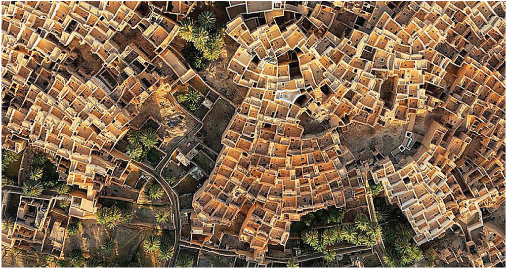
Fig. 1. Closer aerial view with roof terraces.
