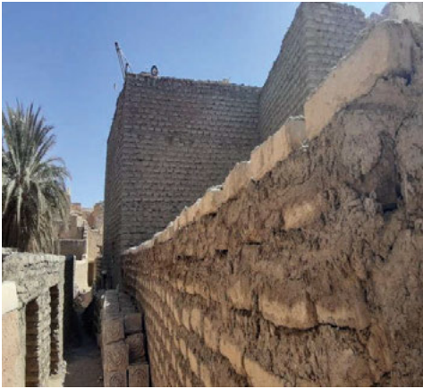
Fig. 10. Reconstruction after disaster.
