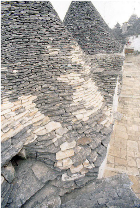
Fig.7. Conservative replacement operation respecting geometric-formal solutions. (Source: Ambrosi, 1990)
