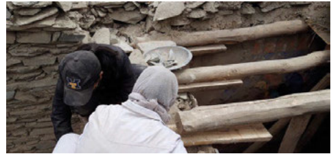
Fig. 17. Placing cantilevers under some of the beams of the entrance hall and fixing them to the stone wall.
