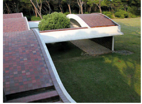
Fig. 3. Cerámicas Cumella: Restoration (2005) of the roofs of La Ricarda by Antoni Bonet. (Source: www.cumella.cat/portfolio/la-ricarda-antoni-bonet )
