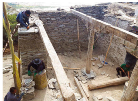
Fig. 8. Reconstruction of the porch with new dry-stone foundations.
