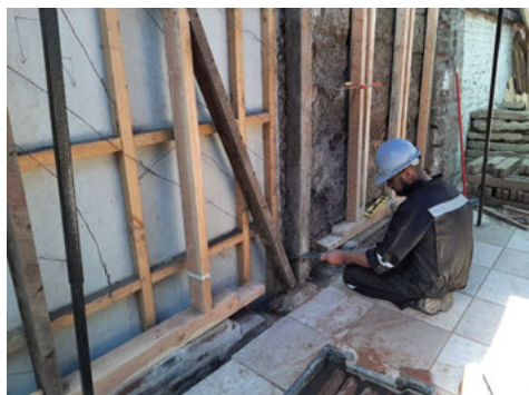
Fig. 7.b. New foundations and retrofitting process in sample (Source: Authors, 2021).
