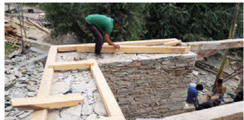
Fig. 18. Insertion of wooden tie beams ( sket shing ).
