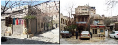
Fig. 6. (right) is the residential structure in one of the Khans, (left) is the usage of the courtyard as parking (Source: Aleppo University's workshop).
