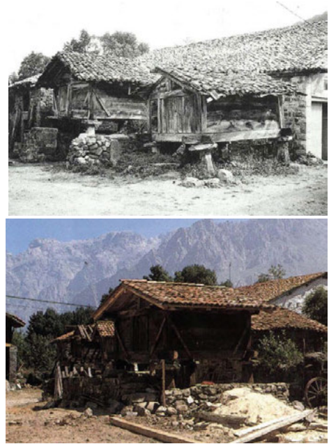
Fig.6. Restoration of one of the hórreos in Valdeón (Luelmo Varela, 1995).
