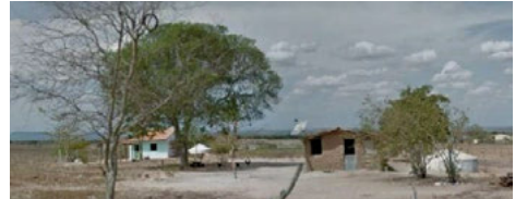
Fig. 2. Example of a wattle-and-daub dwelling in Porto da Folha, Sergipe, Brazil (Source: Google Street View, 2019).
