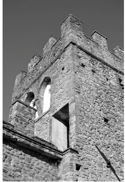
Fig. 4. Well-anchored cornerstones. Tower of the ancient walls in Scarperia (Source: Bordoni., 2021).
