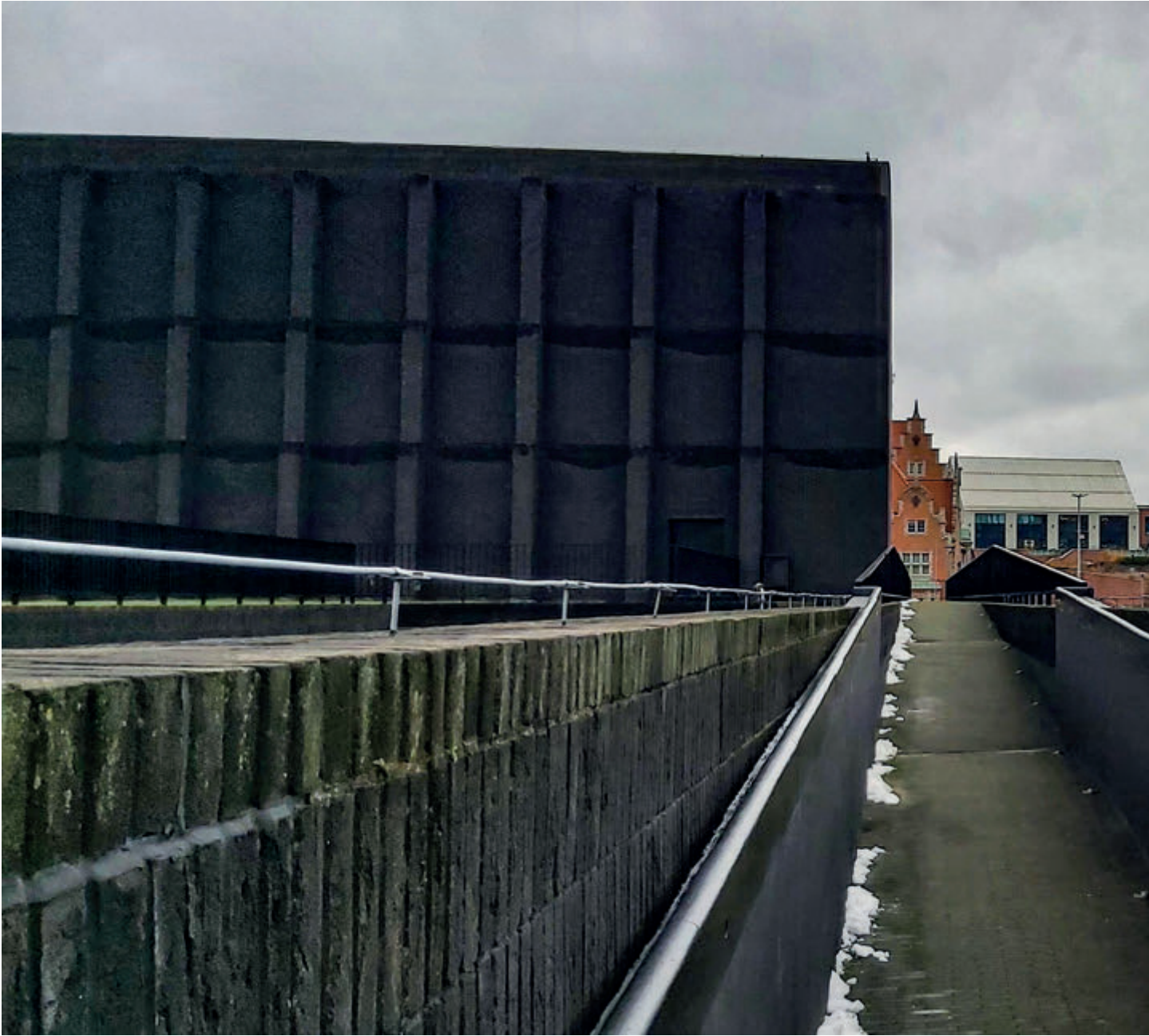
Figure 2 | R. Rizzi, The Shakespearean theatre in Gdańsk, 2005-2014. The perimeter walking system, privileged outpost to overlook the city. Photo: Bahaa Bou Kalfouni.
