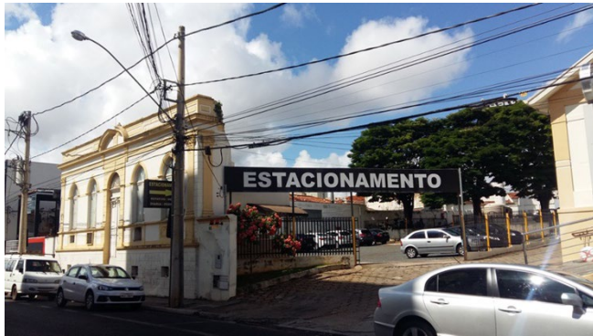
Figure 6 – Building with only the façade preserved – near Rui Barbosa Square. 2019.
