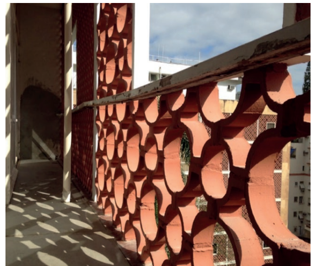
Figure 7 | Balcony railing in cobogó Bristol building, Parque Guinle complex, Rio de Janeiro, Lucio Costa, 1950. © Mara Eskinazi, 2020, with authorization.
