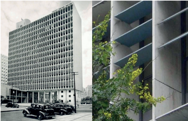
Figures 8 and 9 | (Left) Front façade. Building of Ministry of Education and Health, M.E.S., Rio de Janeiro, Brazil, 1937-1943. Unknown author. (Right) Detail of double-skin façade with movable sunshade louvers in blue fibrocement. Building of Ministry of Education and Health, M.E.S., Rio de Janeiro, Brazil, 1937-1943 © Francisco J. Martinez.
