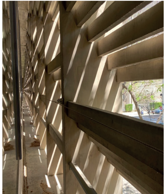
Figures 15 and 16 | (Left) East façade in reinforced concrete with the stepped pattern of the horizontal brise-soleil . The former Law School building. University of Valencia, Moreno Barberà, 1959. (Right) Detail of filtered light into the interior by the outer breathable and perforated skin that overlaps the inner glazed façade. The former Law School building. University of Valencia, Moreno Barberà, 1959. © Photo: Bernardo, Palmero, 2022.
