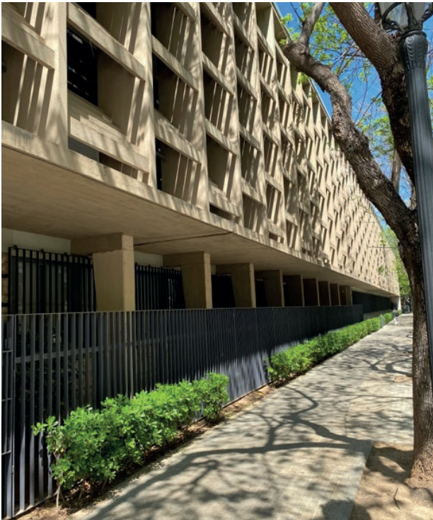
Figures 15 and 16 | (Left) East façade in reinforced concrete with the stepped pattern of the horizontal brise-soleil . The former Law School building. University of Valencia, Moreno Barberà, 1959. (Right) Detail of filtered light into the interior by the outer breathable and perforated skin that overlaps the inner glazed façade. The former Law School building. University of Valencia, Moreno Barberà, 1959. © Photo: Bernardo, Palmero, 2022.
