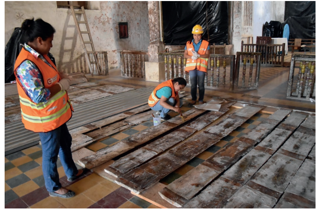
Fig. 1. Local volunteers protecting the interior polychrome wood paneling of the church of San Manuel Colohete. Source: Ferrando et al. 2022.
