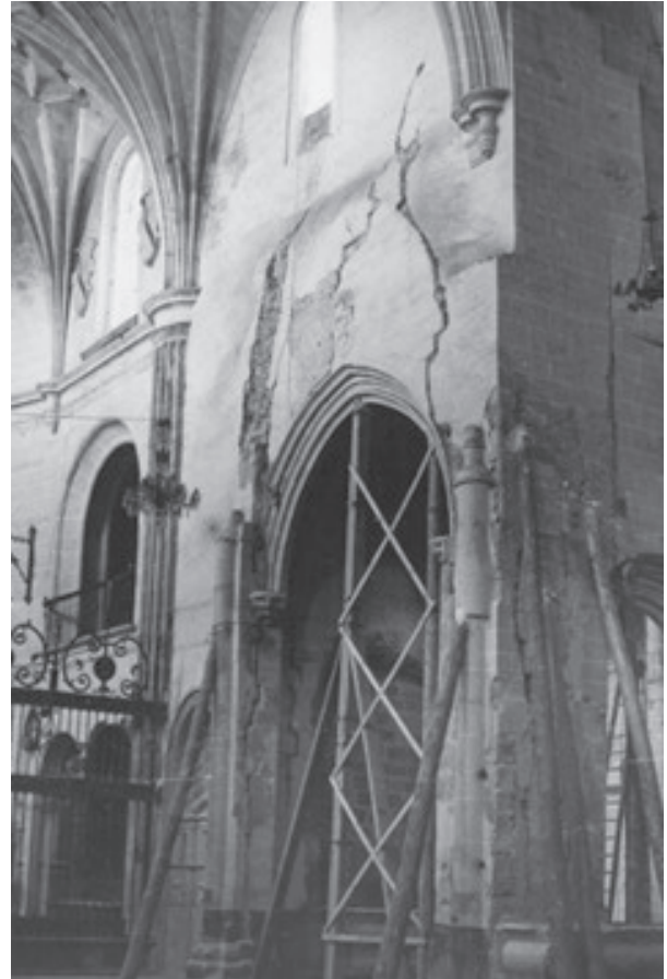
Fig. 3. Photo during the construction in 1948 (Fernández & Hipólito 2013).
