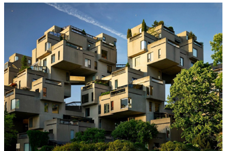
Figure 1. Moshe Safdie, Habitat '67 in Montreal. Source: (Safdie Architects)
