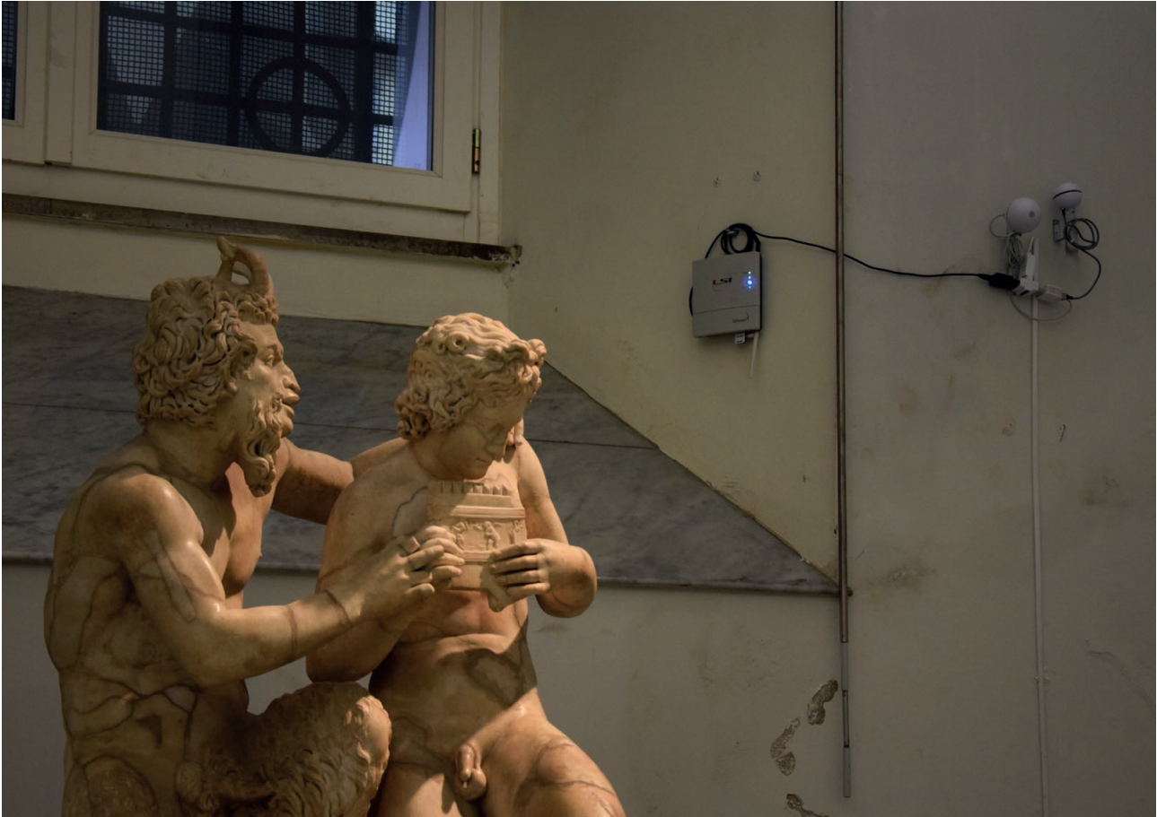
Figure 6 | View of the south windowed wall towards Piazza Museo: the LSI sensors installed for the CapsulART research are visible at the top right. In the wall thickness there is a radio repeater that allows easier interconnection of the monitoring system, which is also connected to the wi-fi network. The system was designed and set up to allow data to be consulted remotely.
