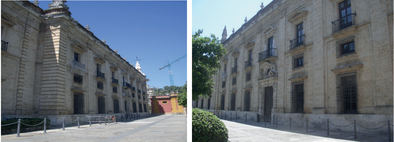
Fig. 2. Facades and access to spaces designed for the homes of the Bosses and Superintendent of the factory. Source: Authors.
