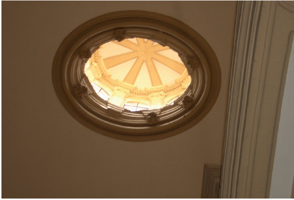
Fig. 3.a. Lanterns designed by Sebastián Van der Borch for light entry into the manufacturing plant. Source: Authors' own creation.
