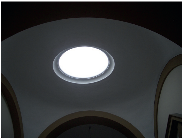
Fig. 3.b. Lanterns designed by Sebastián Van der Borch for light entry into the manufacturing plant. Source: Authors' own creation.
