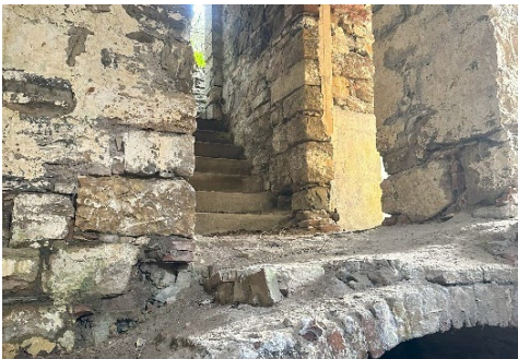
Fig. 6- One of the staircases inside the fortress connecting the lower passages and rooms with the upper levels (Marinaro, 2023).
