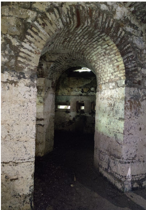
Fig. 11- View of the inside towards the western side (Verdiani, 2023).
