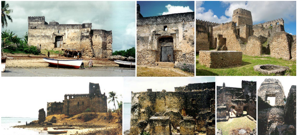
Fig. 7- Several aspects of the condition of the ruins of Kilwa Portuguese-Swahili Fort. (Photos by the Author)
