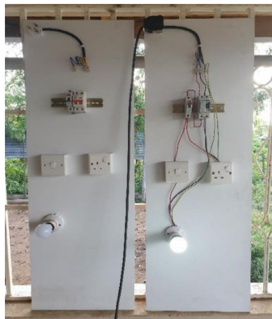
Fig. 4 – Learners during a practical lesson on domestic electrical wiring, boards before & after the practical
