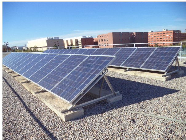
Fig. 1 – Initial photovoltaic installation
