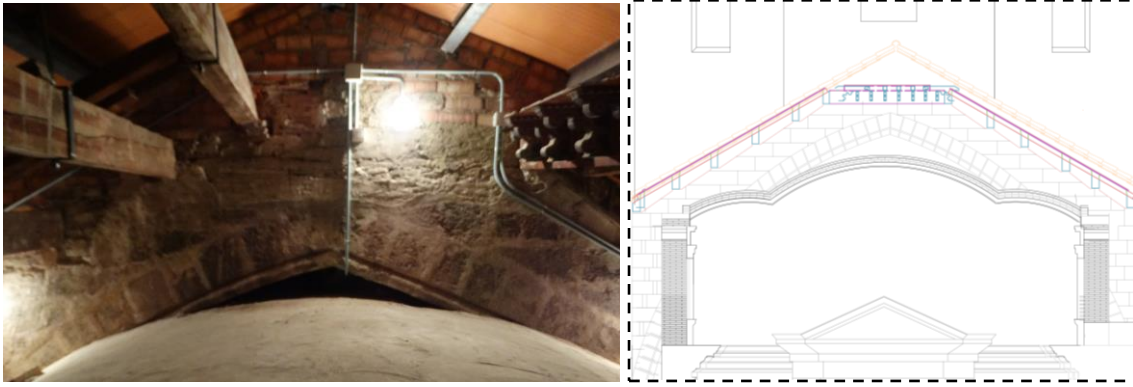
Figure 9: Remaining space in the first bay. Source: Blanco Estévez (2022).
