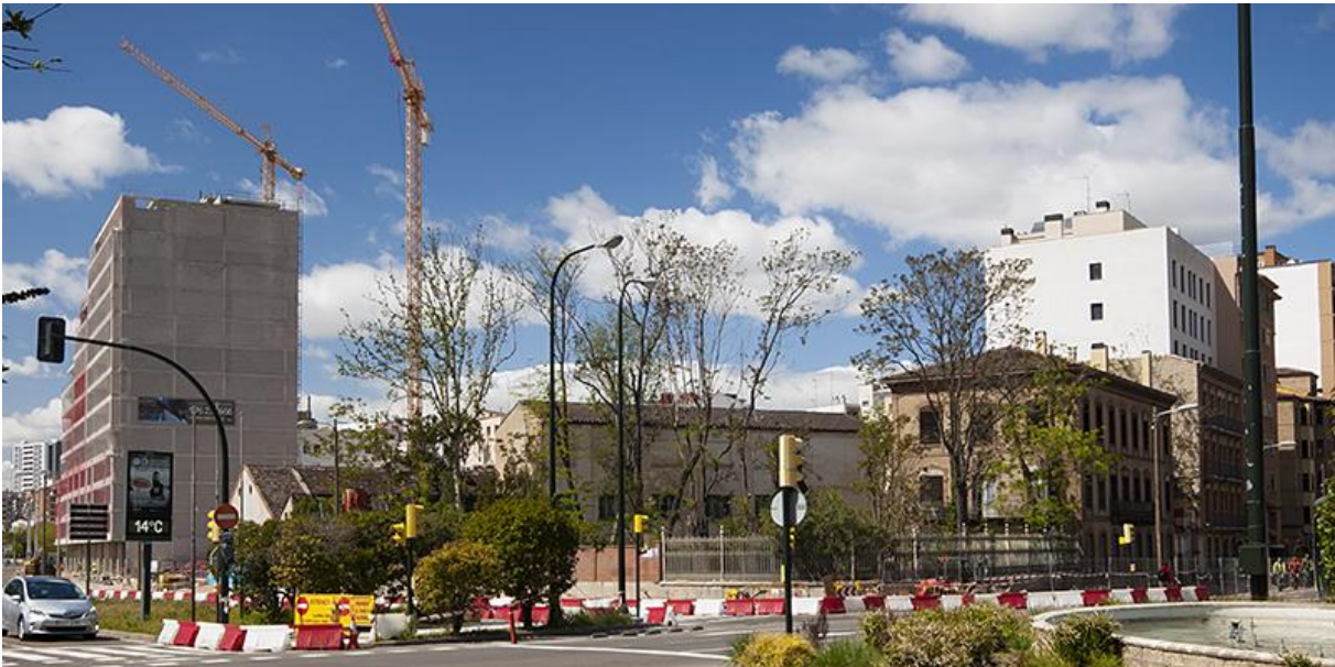
Figure 9. Current view of the Avery foundry among the rubble and the new block of flats under construction. Author: Antonio Duaso Clusa.
