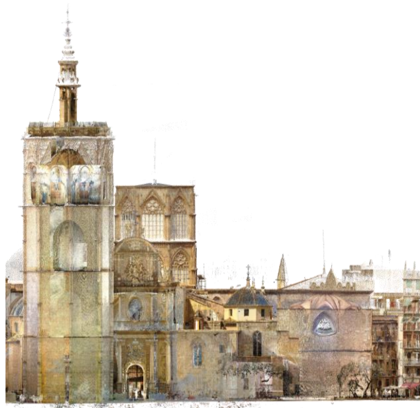
Figure 5. Orthophoto of the Cathedral's baroque facade extracted from the point cloud. Source: Escudero, P.A.
