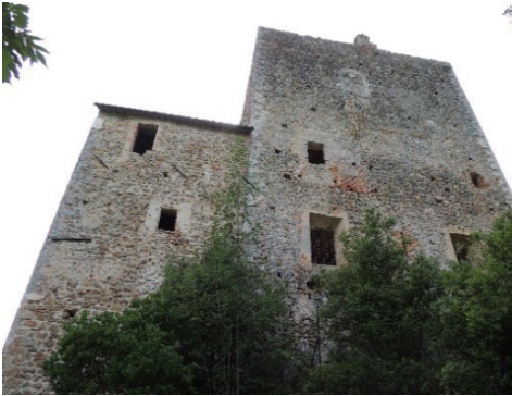
Fig. 4- The north façade of the summit area with the evident resting of the second-period tower to the left (CF2) on the older tower (CF1) to the right (photo by F. Fratini)
