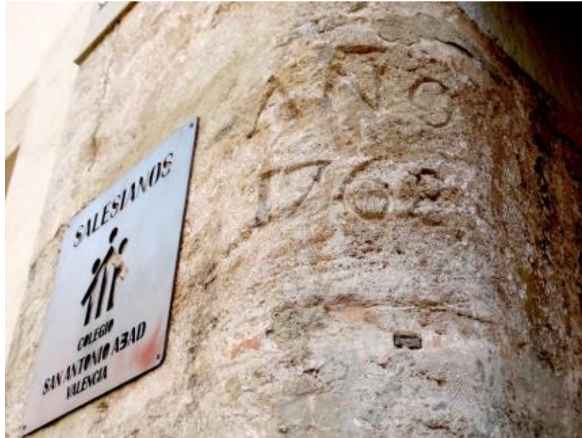
Figure 6: Corner of the outer facade of the cloister. Source: Blanco Estévez (2022).
