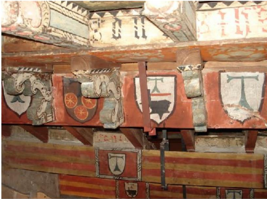
Figure 4: Detail of the roof at present. Source: Blanco Estévez (2022).
