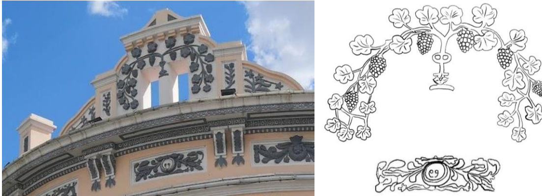
Figure 6. Pattern on the parapet wall and drawing pattern (Author, 2019)
