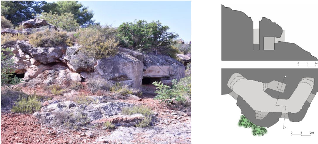
Figure 6 - 7. Pillbox mine-type. Source: own work (2020).
