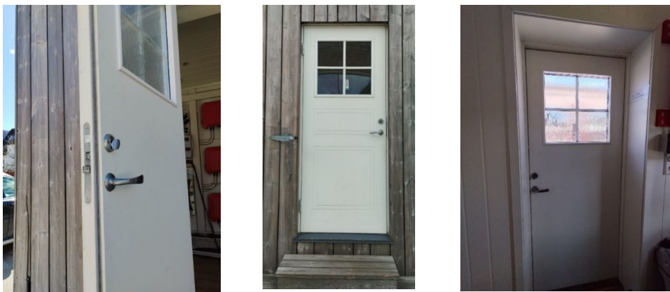
Figure 6. Image SolarLab's entrance door, of own authorship
