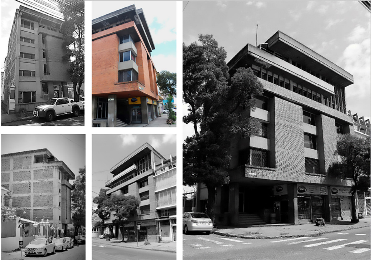
Fig. 6. Photographs of the exterior of the Condominio Profesional building (Source: author, 2024).
