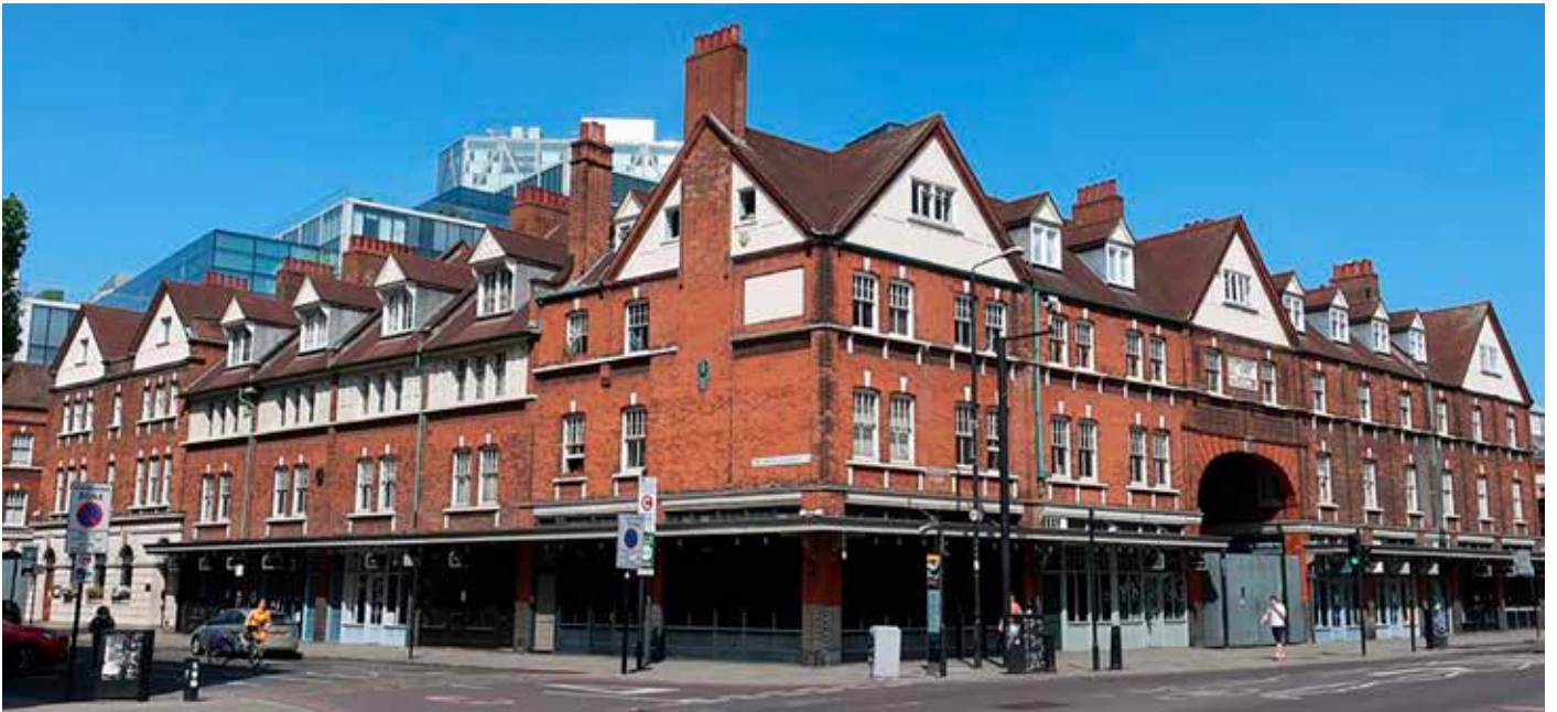
4. La amplia fachada de Spitalfields Old Fruit and Vegetable market. (Fuente: USM). 4. The wide façade of the Spitalfields old Fruit and Vegetable market (pict. by USM).
