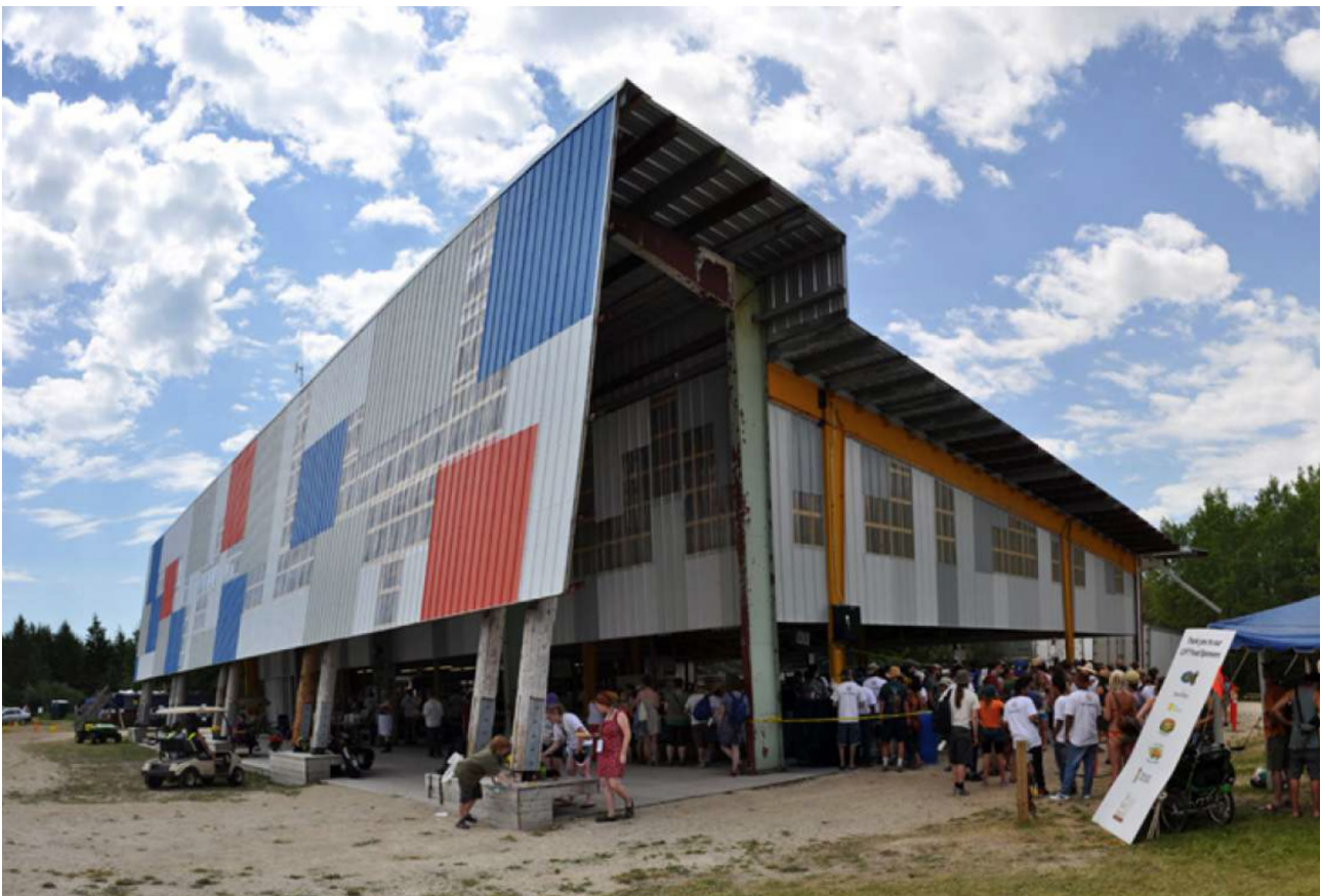
Figure 4 | The building constructed with salvaged steel (Monteyne Architecture, 2011).
