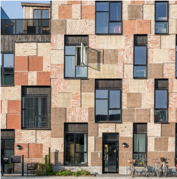
Figure 1 | Reused brick wall pieces for a new façade (Lendager Architecture, 2020).
