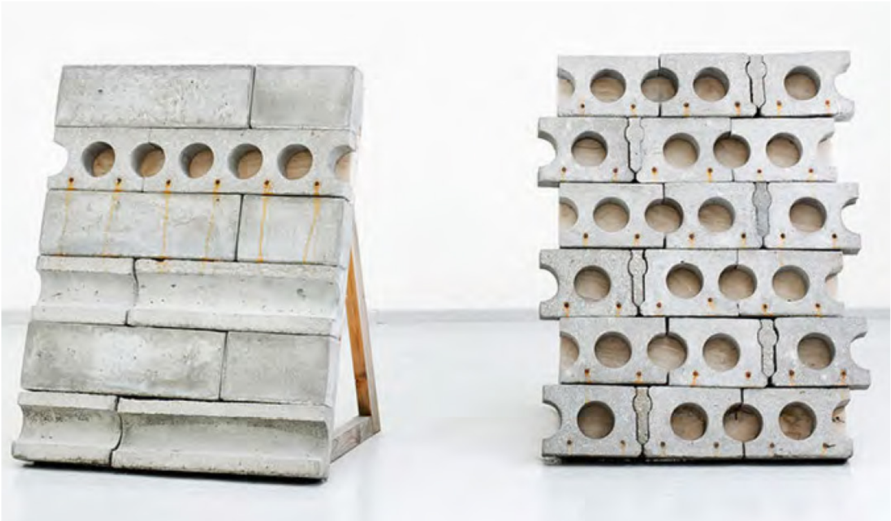
Figure 2 | Precast concrete slabs modified for repurposing as façade elements (Vandkunsten Architects, 2017).
