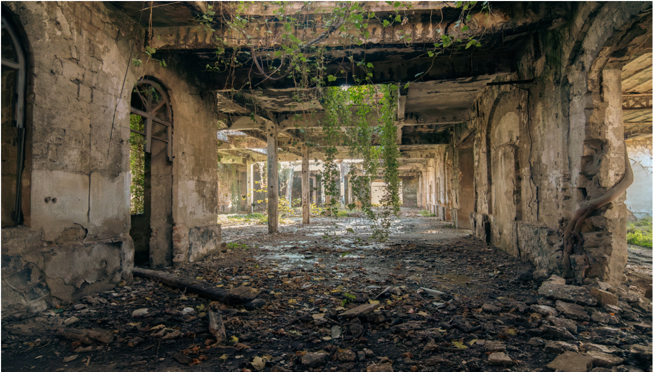
Figure 2 | De Simone factory, interior.
