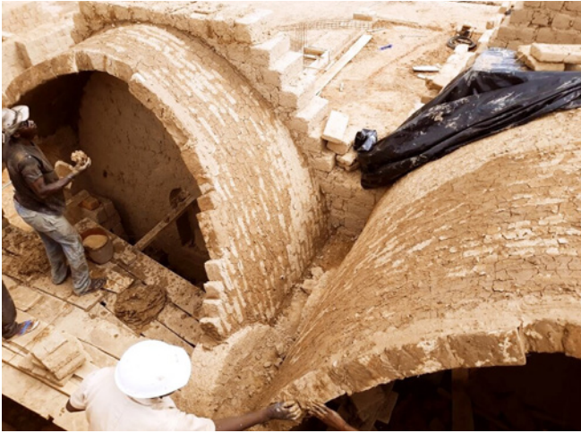
Figure 8. Advances that act as buttresses in https://www.archinea.ch/cites-voutes..
