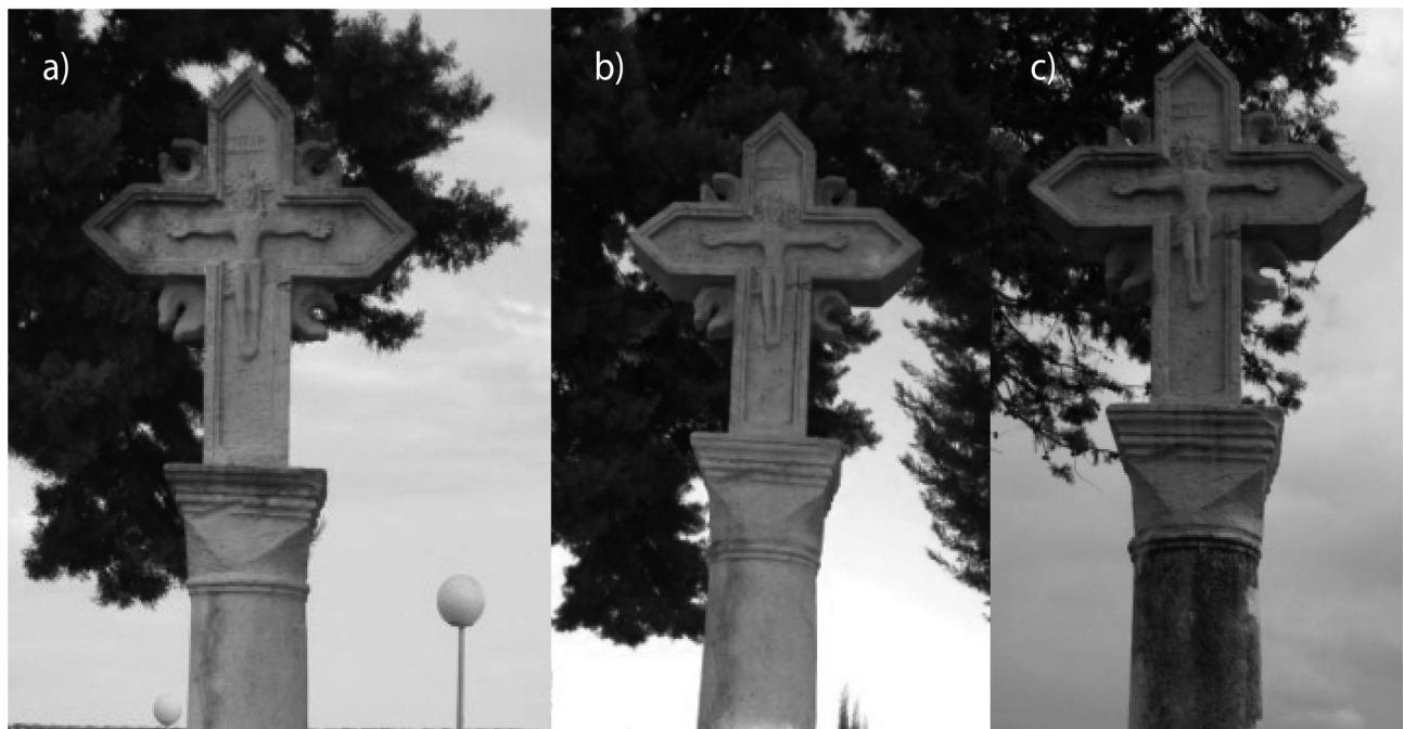
Figure 7. a) Original gothic cross with lichen, b) replica in 2006 and c) replica in 2009. Note: only the cross was replaced, while the column has been retained unchanged. Increase of biological attack of the column whereas the mortar seems not to be affected
