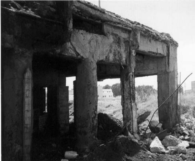
Figure 10. The work platform before intervention
