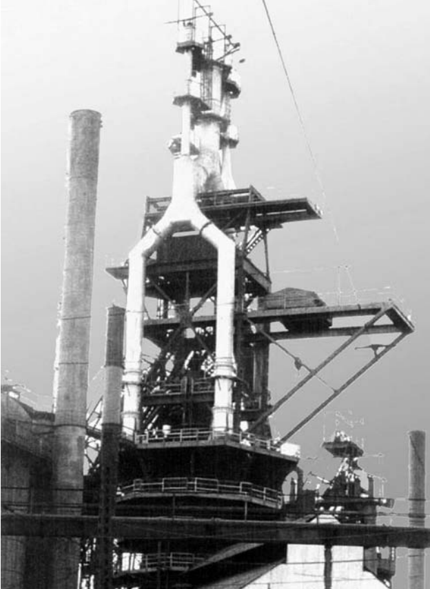
Figure 5. The Number 2 Blast Furnace after rebuilding in 1974. The travellers bestow a characteristic directionality on the whole complex. The colouring of some of the elements can be seen, in particular the safety signs of the handrails
