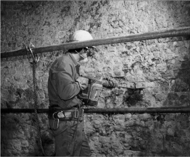
Figure 13. Consolidation work on the refractory coating inside the barrel
