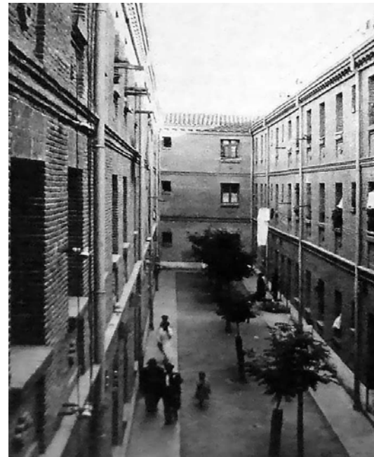
Figure nº016a. Madrid, 1929. View of the interior of the set of 12 group homes with 64 homes qualified as cheap homes, built by 'Constructora Benéfica' in Tenerife and Carlos Rubio streets, Cuatro Caminos neighborhood. Madrid. The houses were double floor in two rows along the sides closed ends forming a courtyard, and were equipped with running water and electricity, gathering few hygienic conditions required by the regulation. Both the houses, as the two schools built as annexes, were planned and supervised by architect Ignacio Aldama y Elorz (sources: Informe sobre la inspección de casas calificadas en la provincia de Madrid, 1925 . Administration General Archive. Caja A.G.A. 2430; and La Construcción Moderna nº 6, 30 March 1922)
