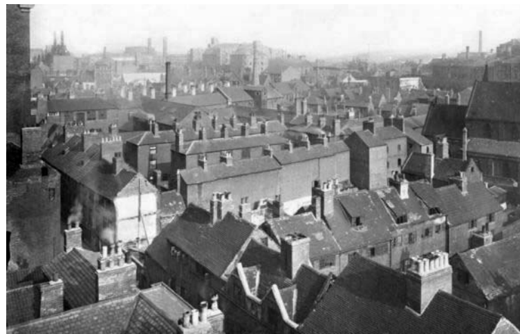
Figure nº 004. Aerial view of densified working class district of Narrow Marsh, Nottingham, 1919. It is possible to distinguish blind-back and back-to back . (source: Nottingham City Council. NTGM001896. Publicada en The History of Working-class Housing . of S.D. Chapman. 1971. p. 198)
