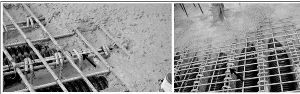
14 15 16 17 18 19 20 21 Figure 2. Embedding in concrete of long-gauge sensors (sensor indicated with arrow). 22
