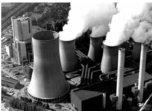
Figure 1: RWE Power Station Niederaussem under construction in 2001 (Photo RWE)
