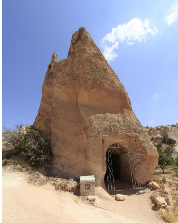
Figure 1: West façade of the Üzümlü Church
