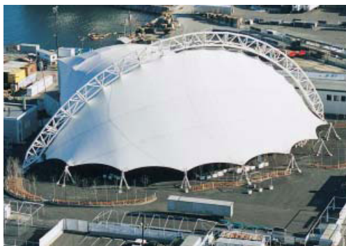
Figure 1: Arch supported tensile roof with conventional, individual suspension cables (Bank of Amerika Pavilion in Boston, MA)
