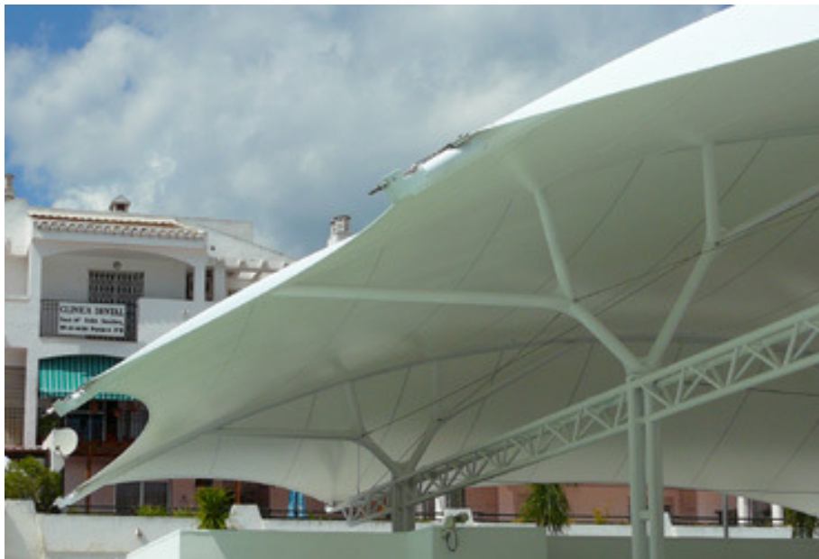
The branches reduce drastically the span of the arches
