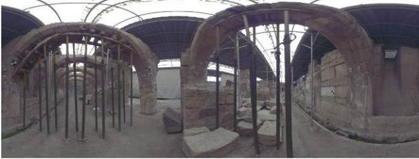
Figure 16: Metal stands to strenght abutments.
