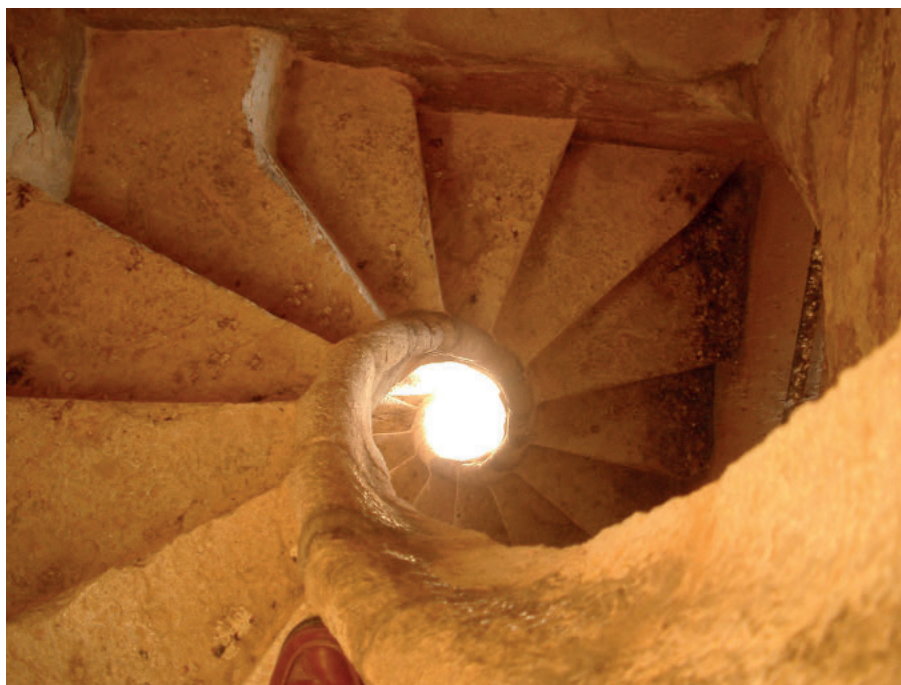
Escalera helicoidal de acceso al campanil Helicoidal staircase of access to the bell tower
