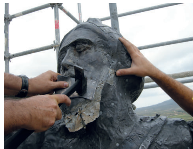
20. Manual application of the lead to the head of the statue of San Juan
