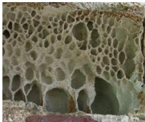
Fig. 6- Alveolation with different size of alveoli (15-80 mm) with lightly iso-orientation, related to different welding inside the same ashlar.
